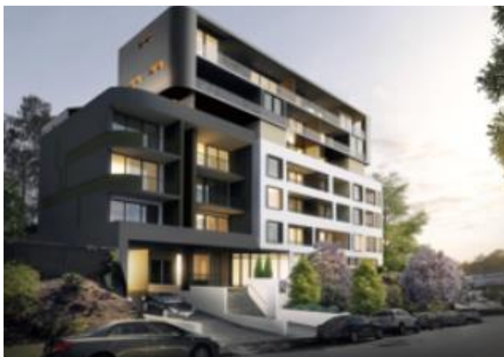
Figure 11 – Approved Development at 1 Ellen Subway, Mortdale
