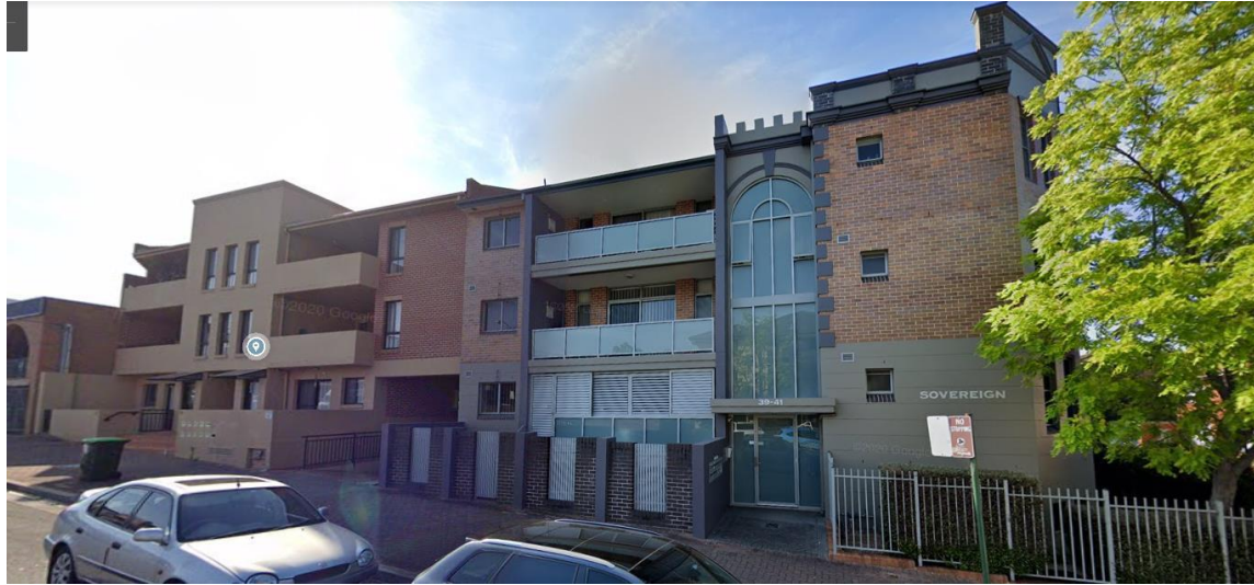
Figure 6 - Existing 3 storey residential development (35-39 Pitt Street, Mortdale)
