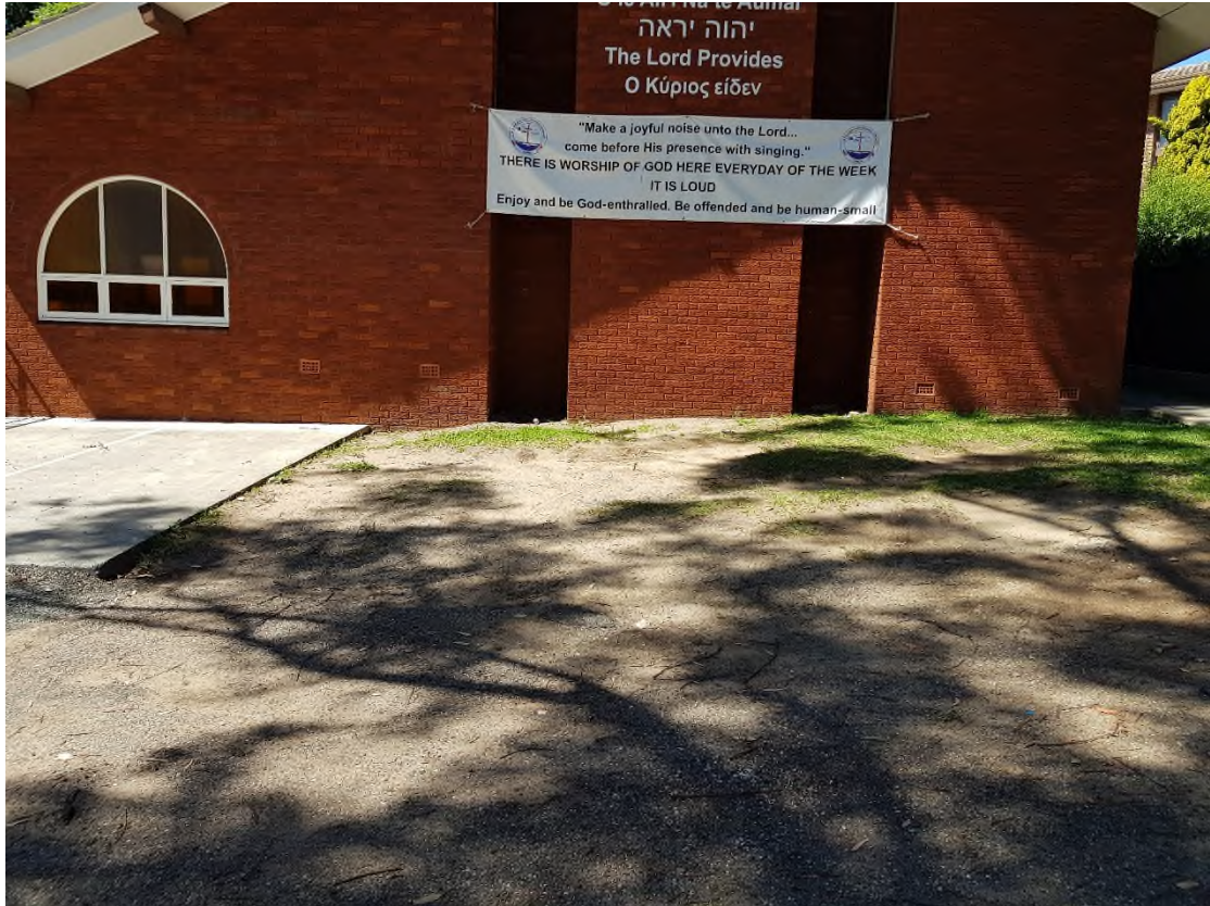
Photograph A3.1: Front of Building
