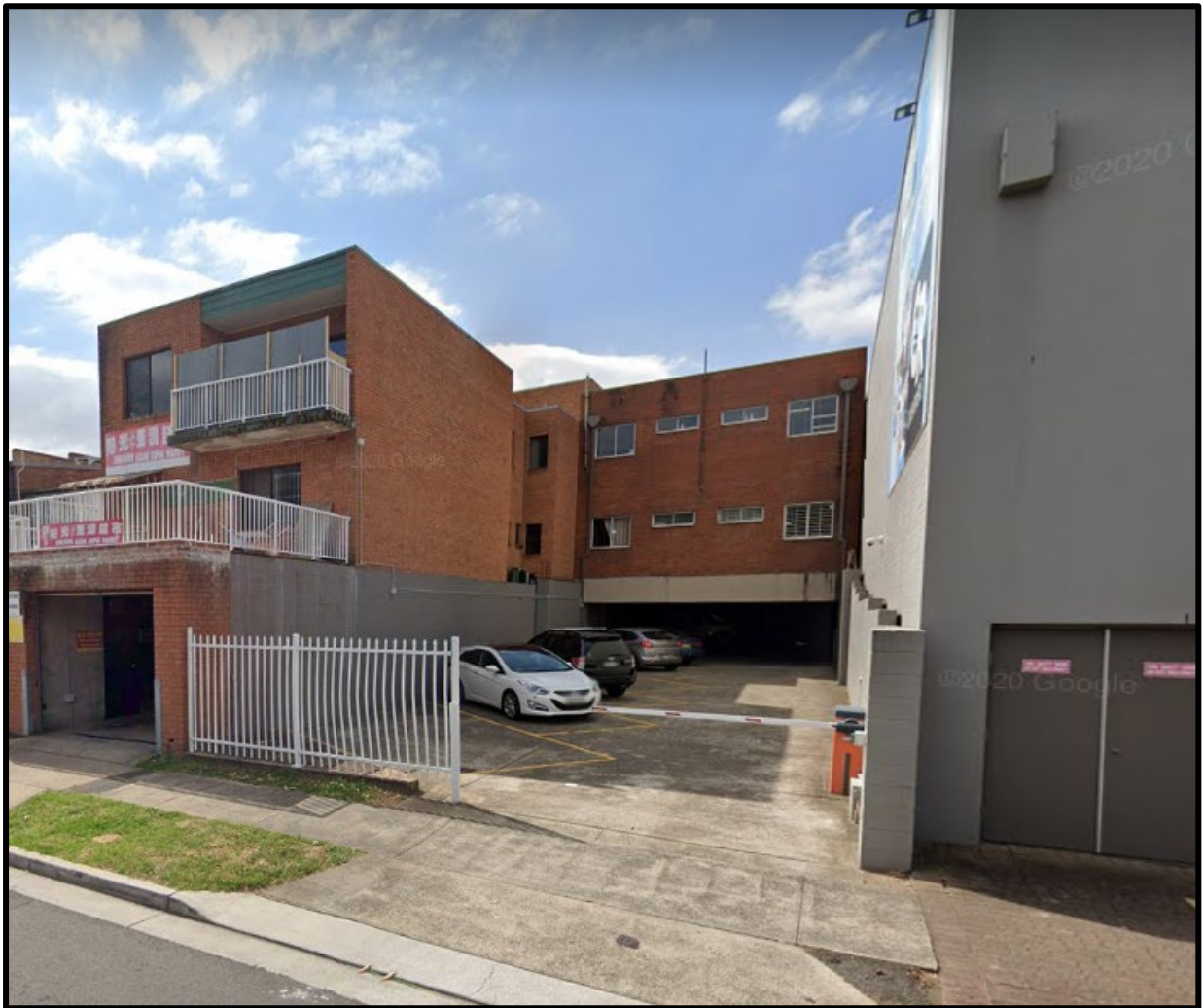
Figure 5: View of location of proposed extension (Littleton Street)
