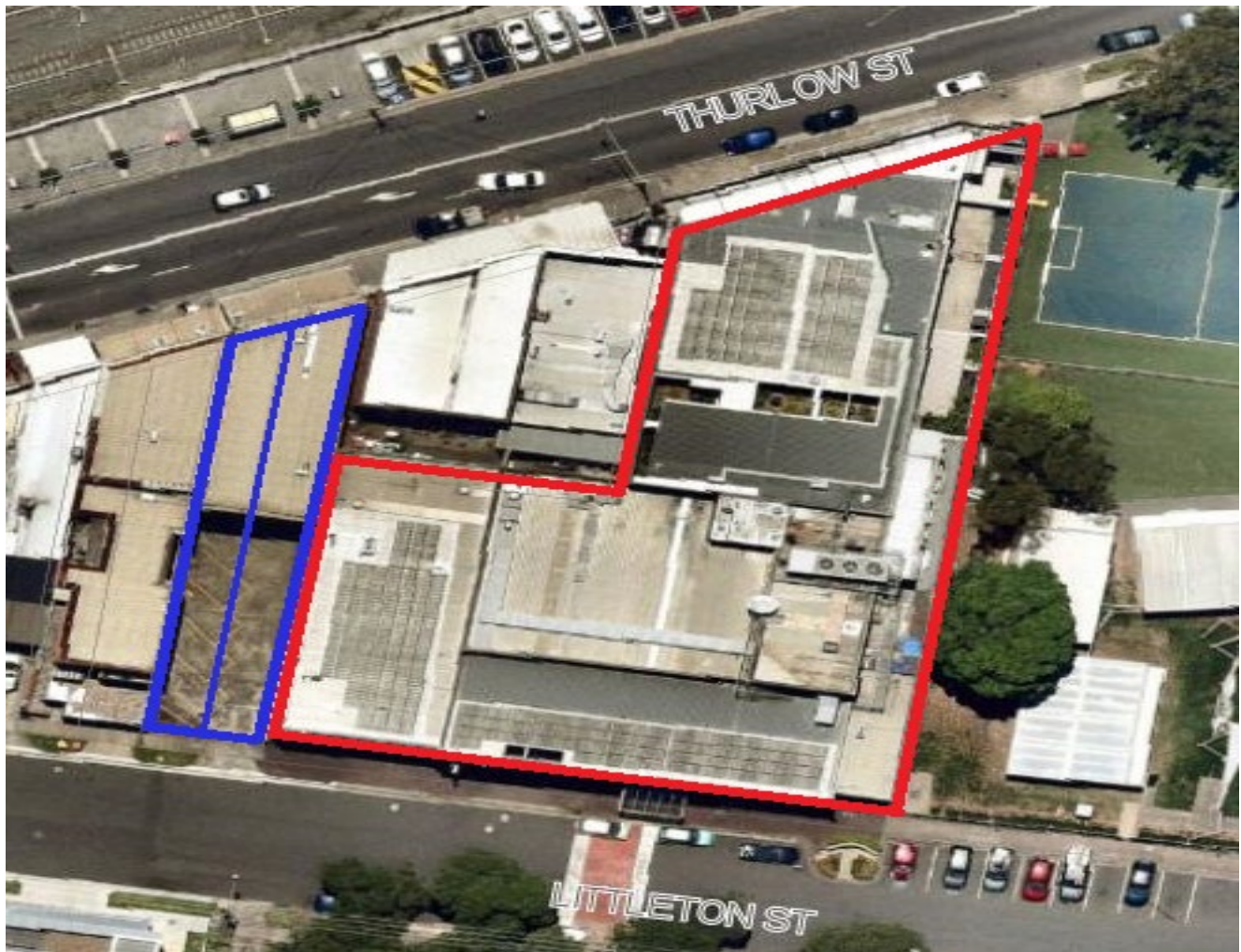
Figure 1: Aerial view of site (club) in red, with proposed location of works (Site) in blue (Source: Intramap 2022 )
