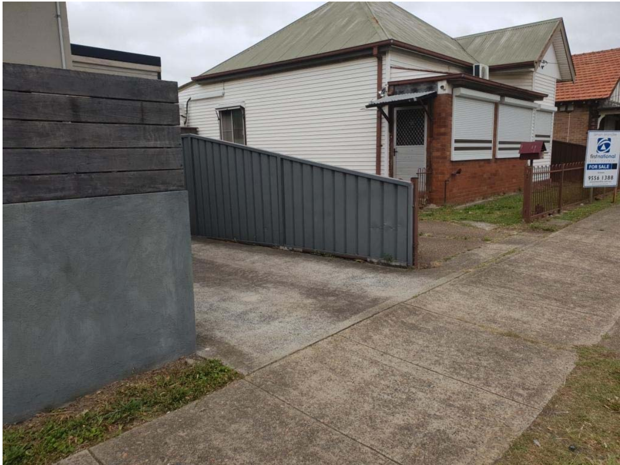
Photograph of existing side fence
