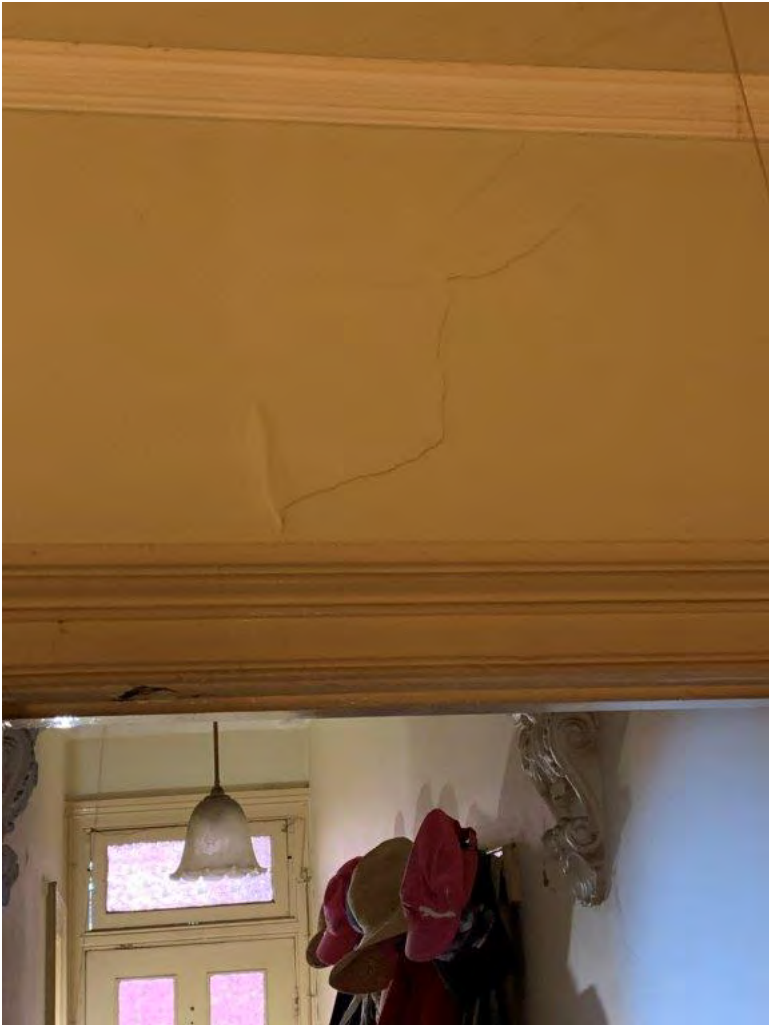
Photo 4 - Cracks in Brick Wall
