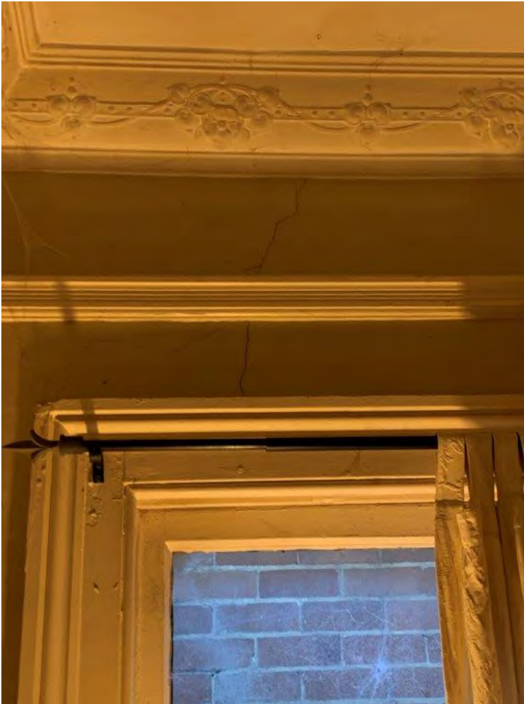
Photo 5 Cracks in Brick Wall
