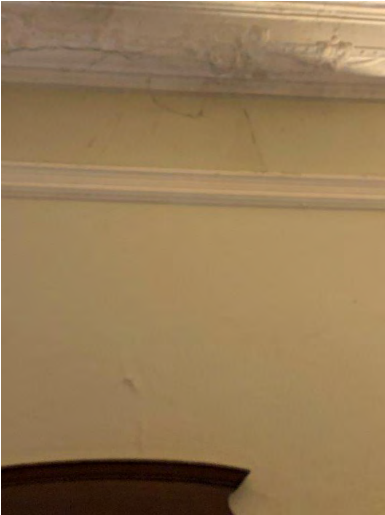
Photo 6 - Cracks in Brick Wall
