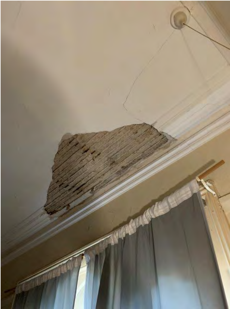
Photo 7 - Cracks in Ceiling and Brick Wall
