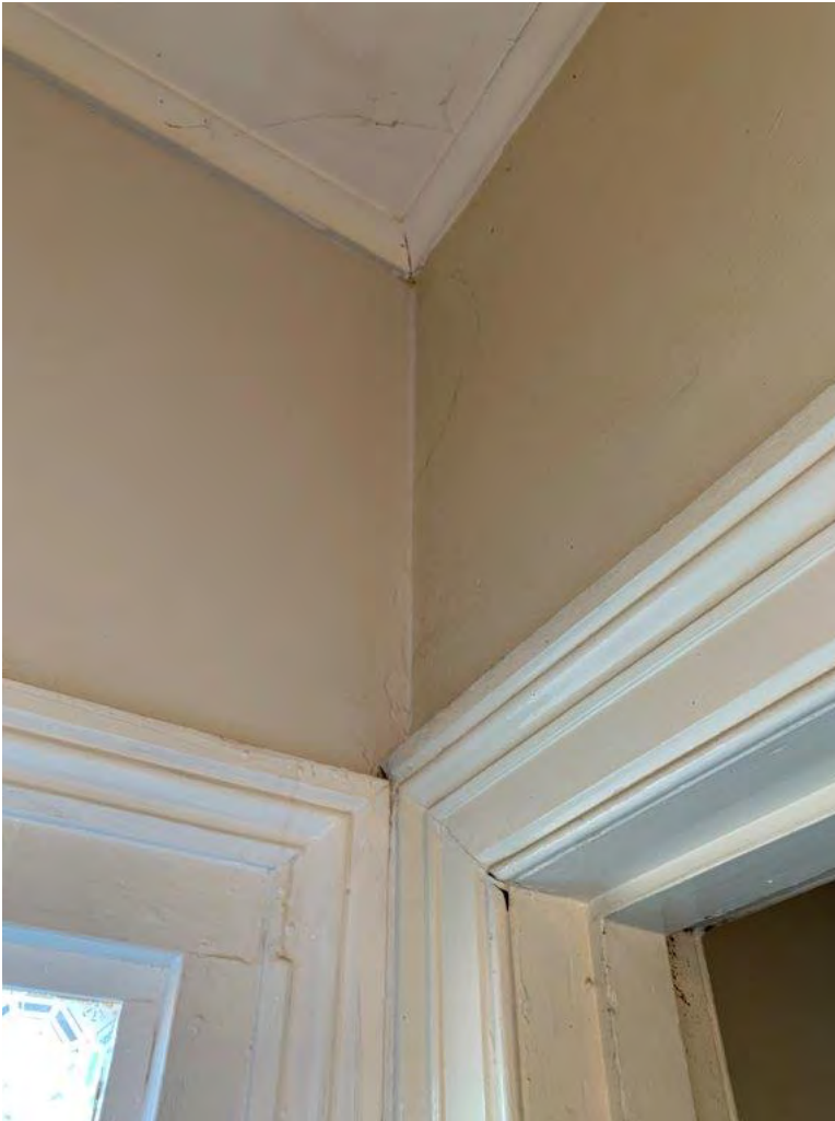
Photo 14 - Cracks in Brick Wall
