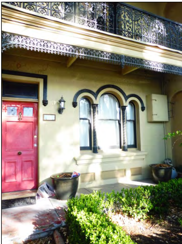
Figure 3.28 Detail of the front façade of No. 14 which retains rendered mouldings on the ground floor façade, however, the first floor cast iron valance is missing.
