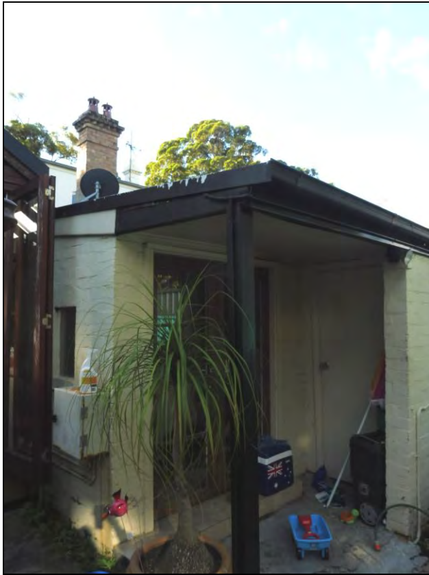
Figure 3.37 The single storey rear wing is also constructed of painted brick. The chimney and small addition remain, however, the openings and roof have been modified.
