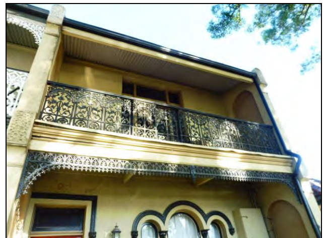
Figure 3.28 Detail of the front façade of No. 14 which retains rendered mouldings on the ground floor façade, however, the first floor cast iron valance is missing.
