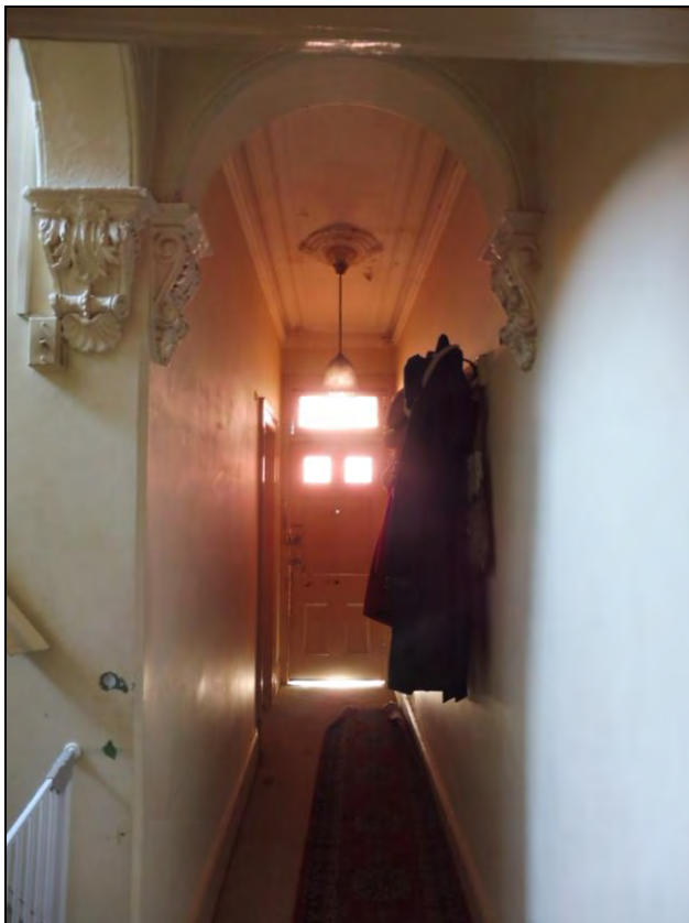
Figure 3.30 The hallway has a high ceiling with decorative plaster cornice and ceiling rose and arch with decorative plaster brackets.
