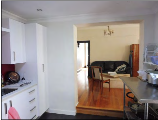
Figure 3.46 A large opening has been made to access the rear wing.
