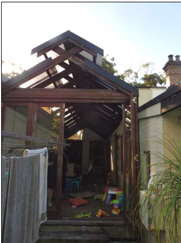
Figure 3.36 The deck and lightweight infill added to the rear setback.
