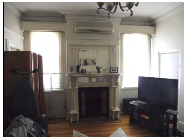
Figure 3.45 The main living room ceiling and floor have been renewed, however, retains the fireplace and early timber joinery.
