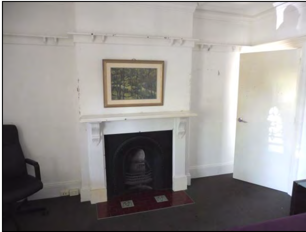
Figure 3.41 The front bedroom retains a fireplace and early timber joinery and high plaster ceiling.
