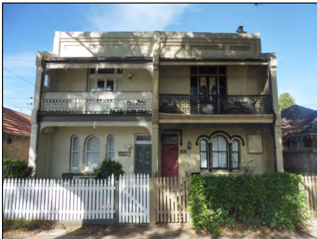
Figure 3.25 The front façades retain their early form details including the high parapet, projecting central party and end walls and associated details, also open front verandahs and balconies, pattern of openings with timber framed windows and doors and most of cast iron lace elements.
