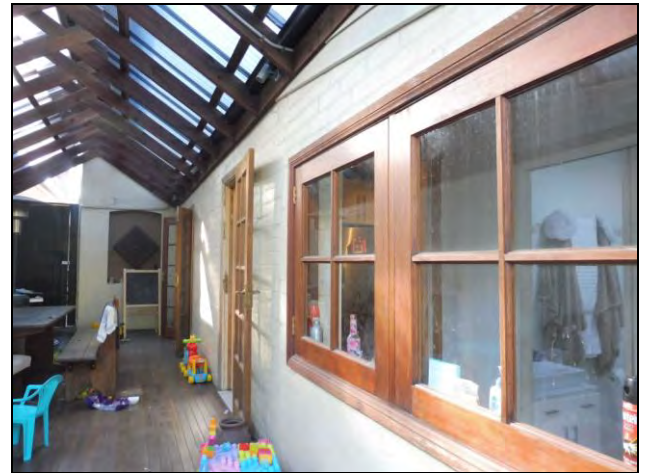
Figure 3.35 A timber deck and lightweight roof have been added to the rear setback of No. 14. The openings have also been modified with new timber framed windows and doors added.
