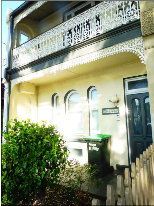
Figure 3.27 Detail of the front façade details of No. 16 which retains the overall form and details, however, the rendered mouldings have been removed from the ground floor façade and a small window has also been added to the blind arch of the the northern end wall on the first floor.
