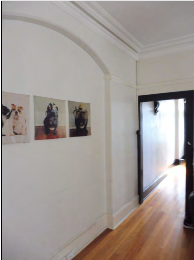
Figure 3.44 The ground floor hall also has blind arches on the central party wall and leads into the main living room.
