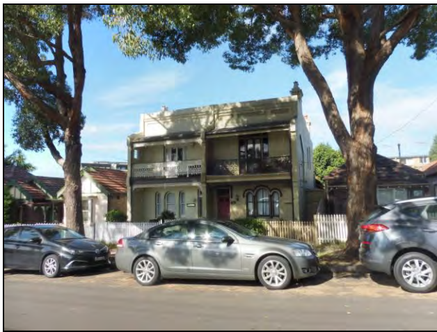
Figure 3.22 Nos. 14 and 16 are a pair of Victorian style dwellings with two storey parapeted main wing and projecting end and central party walls which retain original details and frame open verandah and balconies.
