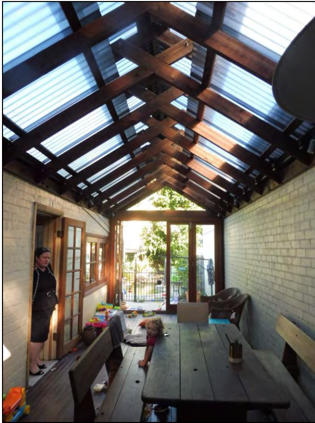
Figure 3.35 A timber deck and lightweight roof have been added to the rear setback of No. 14. The openings have also been modified with new timber framed windows and doors added.
