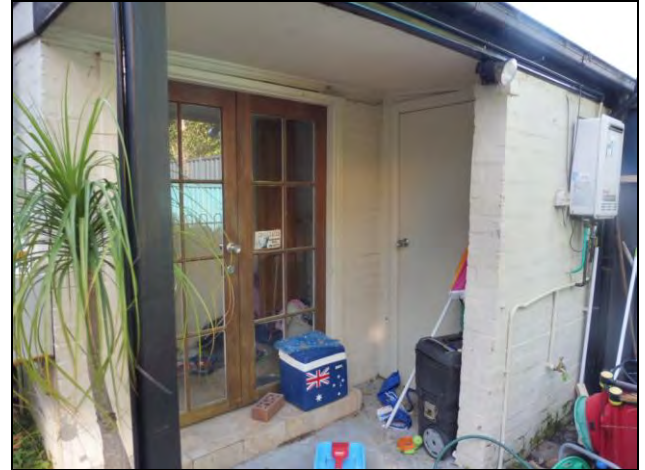
Figure 3.37 The single storey rear wing is also constructed of painted brick. The chimney and small addition remain, however, the openings and roof have been modified.
