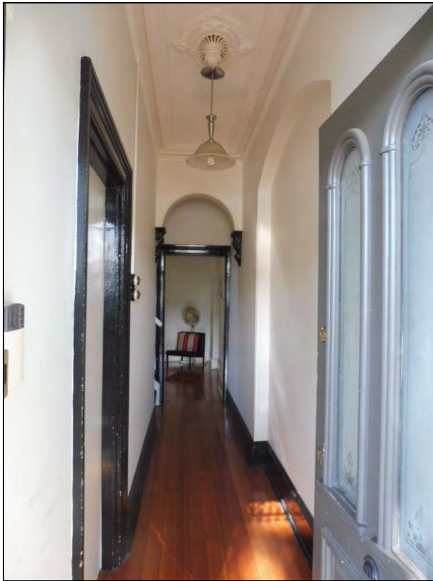
Figure 3.39 The interior of No. 16 also retains typical layout with two rooms on the ground and first floor accessed by a side corridor running along the central party wall. The hallway also has a high ceiling with decorative plaster cornice and ceiling rose and arch with decorative plaster brackets and new timber flooring.
